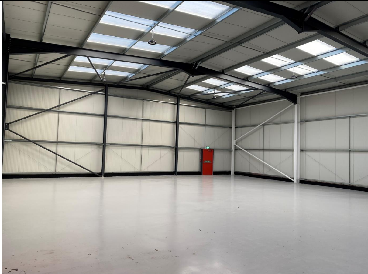
Example view of inside the warehouse
