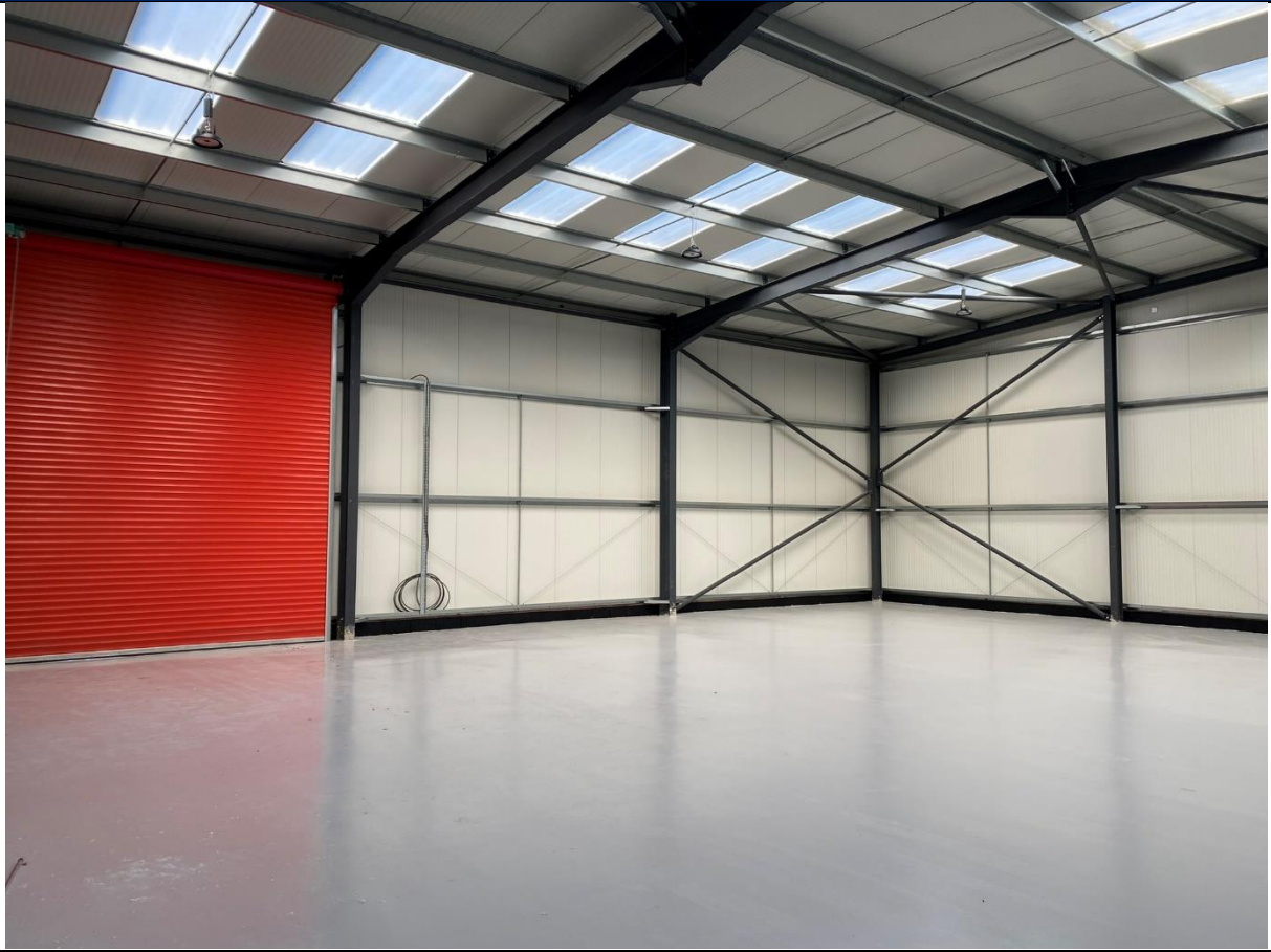
Example view of inside the warehouse
